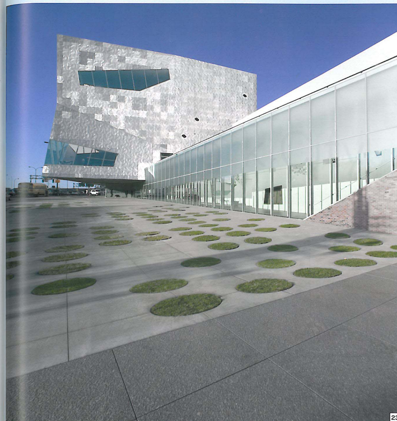
23: Photo of Walker skin taken December 2006 reveals the continuity of surface and apparent variety created through the single metal mesh panel.
